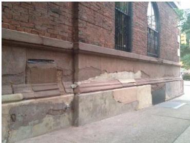
South Elevation Water Table - Before
