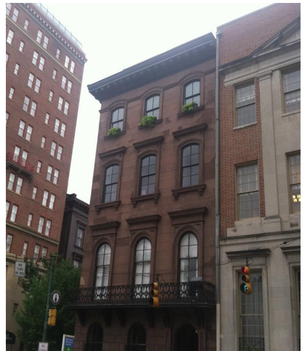
Main Elevation After Restoration
