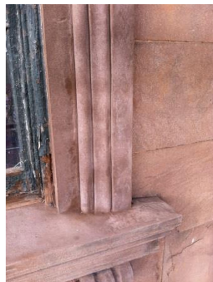
Window Jamb - After
