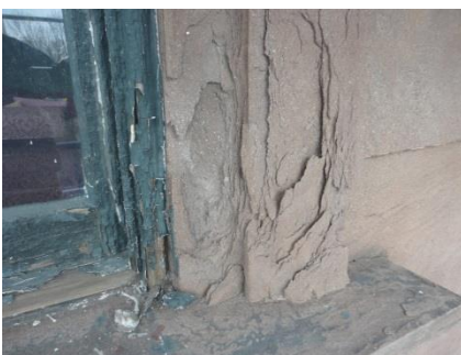
Window Jamb - Before
