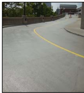
South Garage Ramp Phase 1 Base Coat
