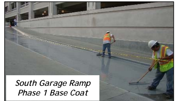
Lower Ramp at 4 th floor Coating over Beam Line
