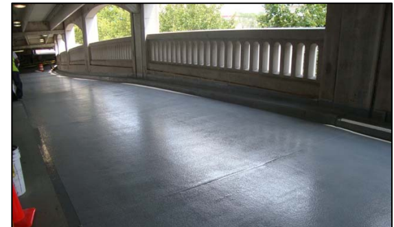
South Garage Ramp Phase 1 Base Coat
