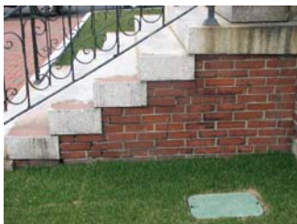
Entrance Masonry & Steps Before
