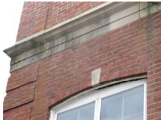
Masonry Arch Before
