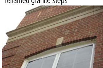
Re-built Masonry Arch - After
