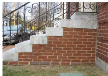
Repointed masonry, cleaned & re-flamed granite steps
