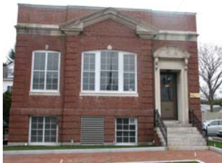
Front Elevation Before
