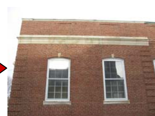
Repaired & Cleaned Masonry
