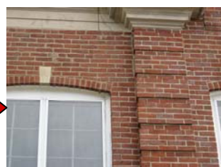
Cleaned Limestone & Masonry
