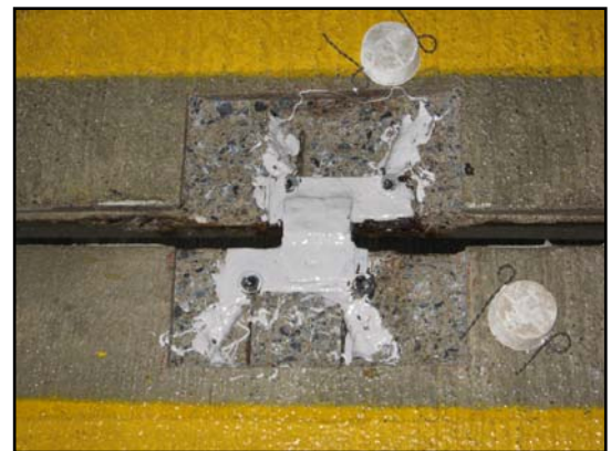
Newly prepared Double-T Connection with zinc anodes ready for installation
