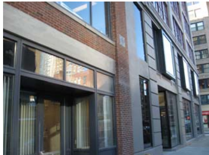
New façade at Kneeland St. Entrance
